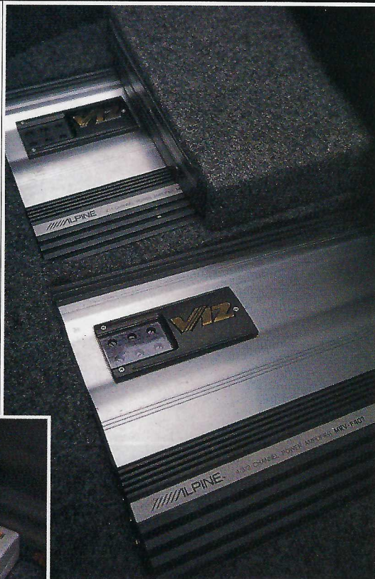
TOYS IN THE TRUNK: Two Alpine amps are sunk into a panel that fits over the trunk floor (above); an Alpine CD changer sits on top of one of the amps in a custom housing (left).
