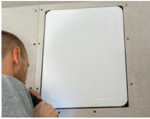
Edge5 speaker installed in the wall awaiting compound and paint.
