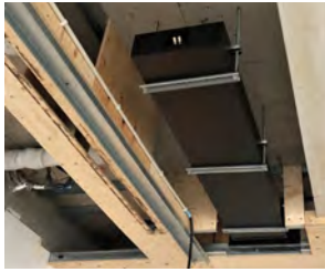
The sizable Amina ALF120 subwoofer secured above the ceiling.
