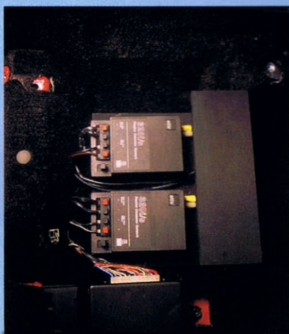
Crossovers and amp each have a shroud made of MDF to protect them from back-seat passengers' feet.
