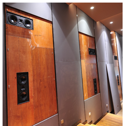
Side panels under construction housing James Loudspeaker QX630 speakers with Quad Tweeter
