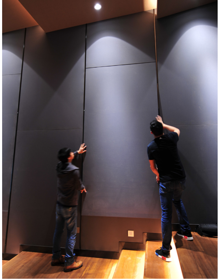
Acoustic panels being set into place
