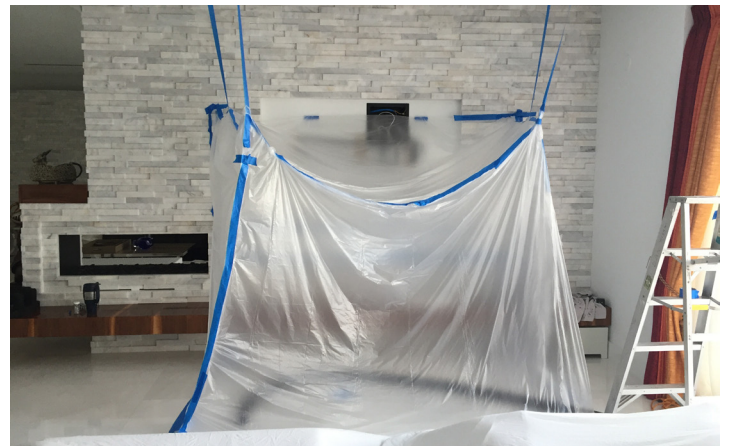
The mason tented off the room as they precisely ground the marble around the opening for the sound bar
